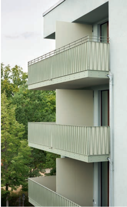
Kopfbau | Head-end building
